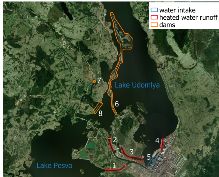
Figure 2. Location of the main hydraulic structures in the cooling lakes of the Kalinin NPP: 1 – water discharge through the canal into the lake Pesvo; 2 – water discharge through the canal into the lake Udomlya; 3 – outlet channel of cooling towers 1,2; 4 – outlet channel of cooling towers 3,4; 5 – water intake; 6 – dam directing the flow of heated waters in Lake Udomlya; 7 – dam on the river Syezha; 8 – dam directing the flow of water at the source of the river Syezha.
