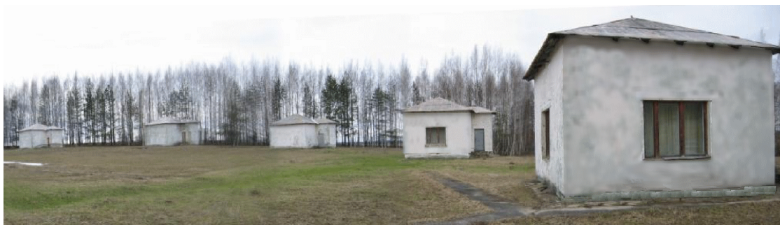
Figure 2. Pavilions dedicated to electric and magnetic measurements in Borok Geophysical Observatory. The absolute house is the first from the right and the variation room is the first from the left.
