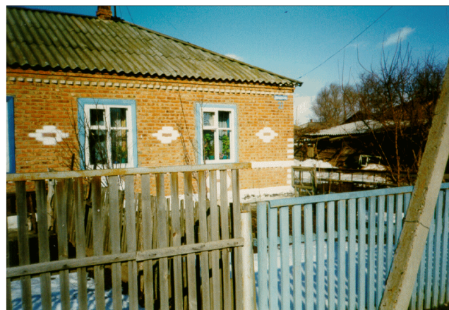
Figure 4. Typical country house (Village Volochaevskaya). It is a predominant type of buildings: one store good quality brick with cement mortar. Basis is square or slightly elongated.
